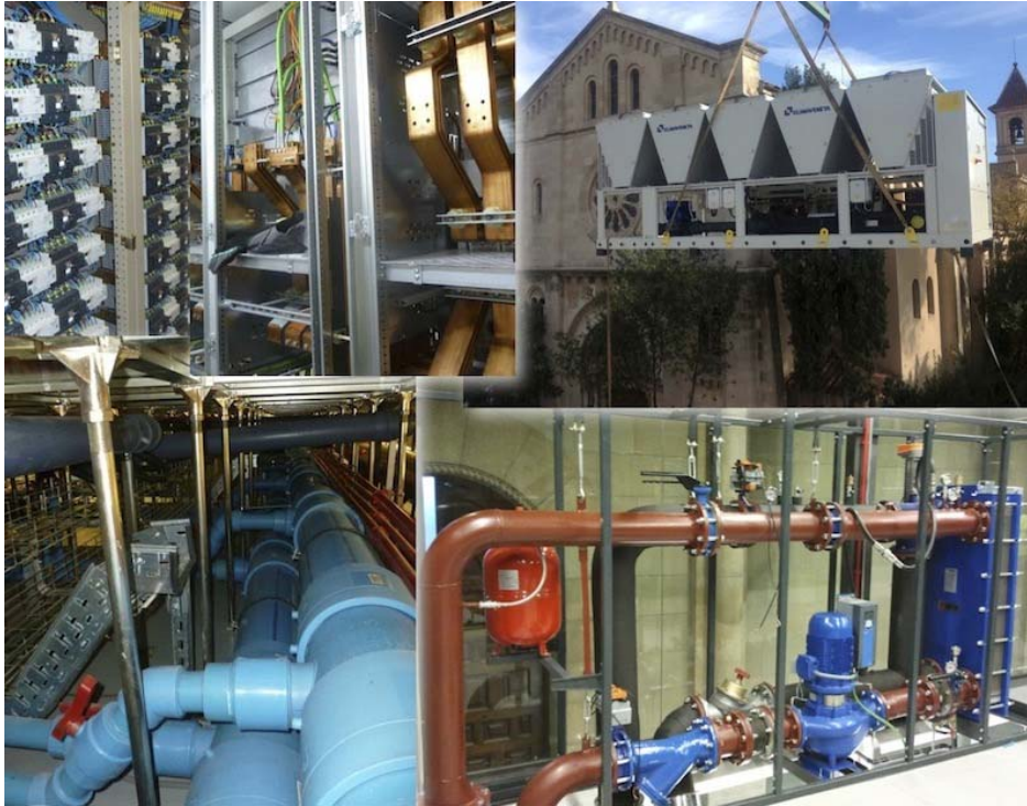
Figure 2: Pictures taken during the site preparation
